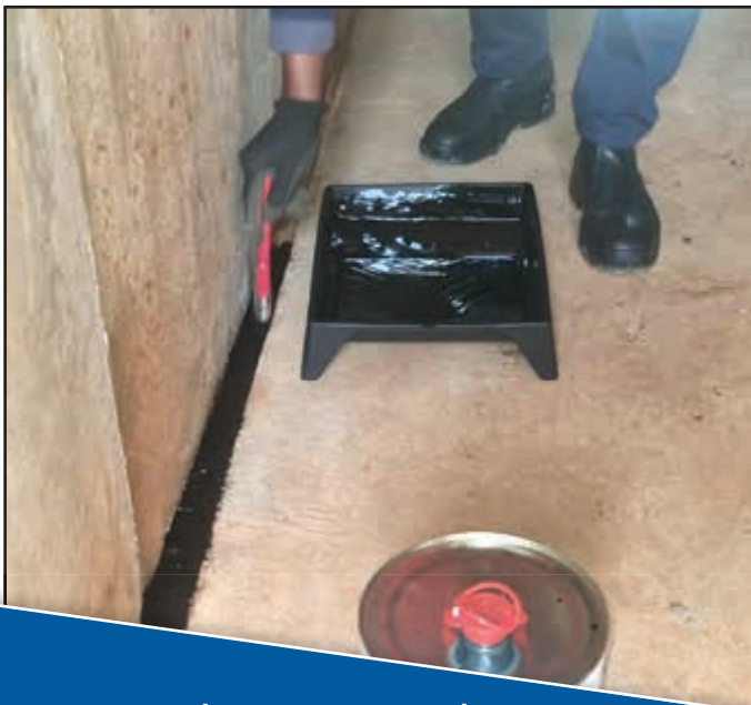
Denso Primer D™ and Denso™ Joint Sealer being applied on the inside of the culverts that have already been stacked.
