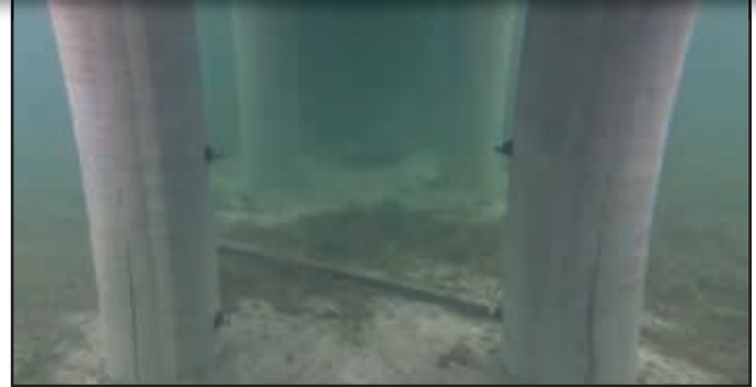
Underwater view of the completed SeaShield 400™ System.
