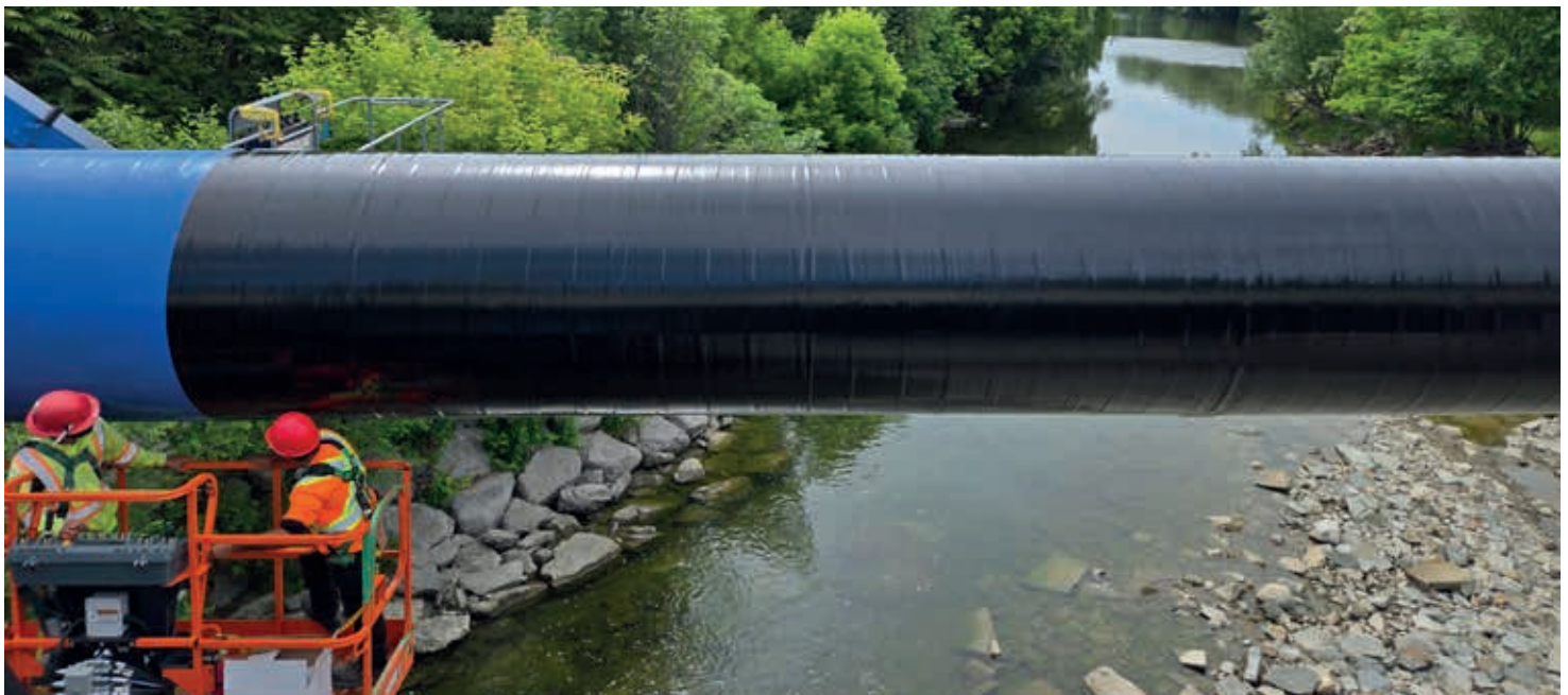
Below: A wrap of ViscoWrap™ PE Outerwrap completes the protective system.
