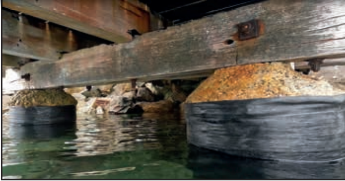
The completed SeaShield 70™ System.
