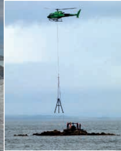
The new light structure being airlifted into place by helicopter.
