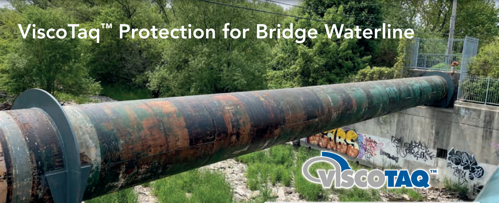
The bridge waterline cleaned and ready for the Viscotaq System.
