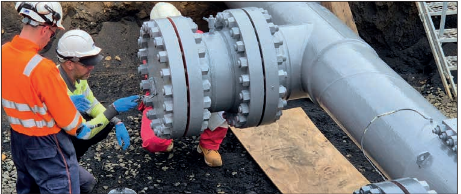
Above: Protal 7300 (UK) can be applied to dry, damp or wet surfaces. Below: Protal 7300 (UK) can be applied by roller, brush or pad.
