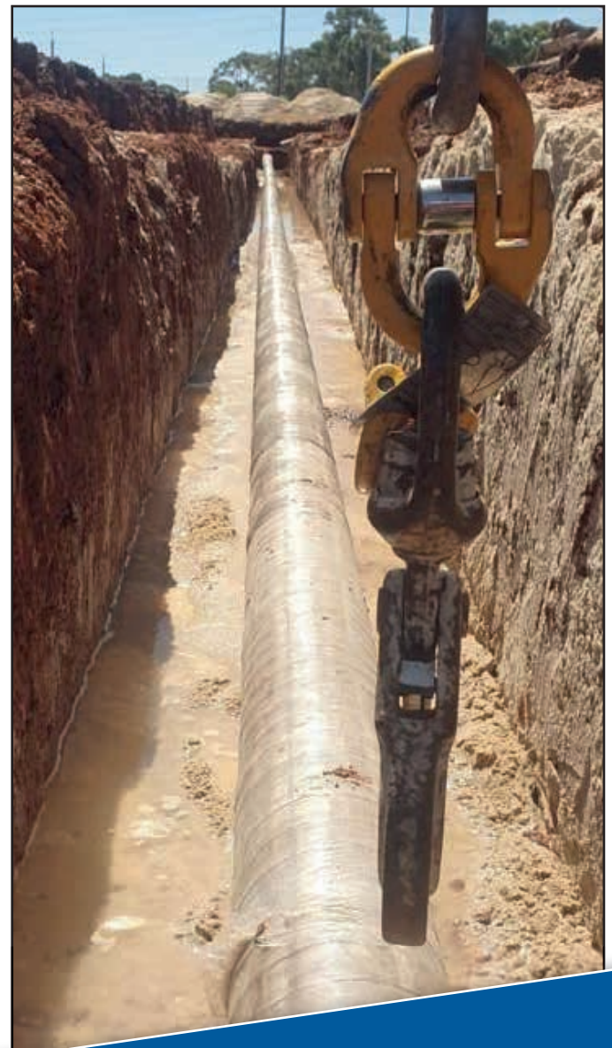
Below: The Bore-wrap protected pipe is lowered into position so that the drilling can begin.
