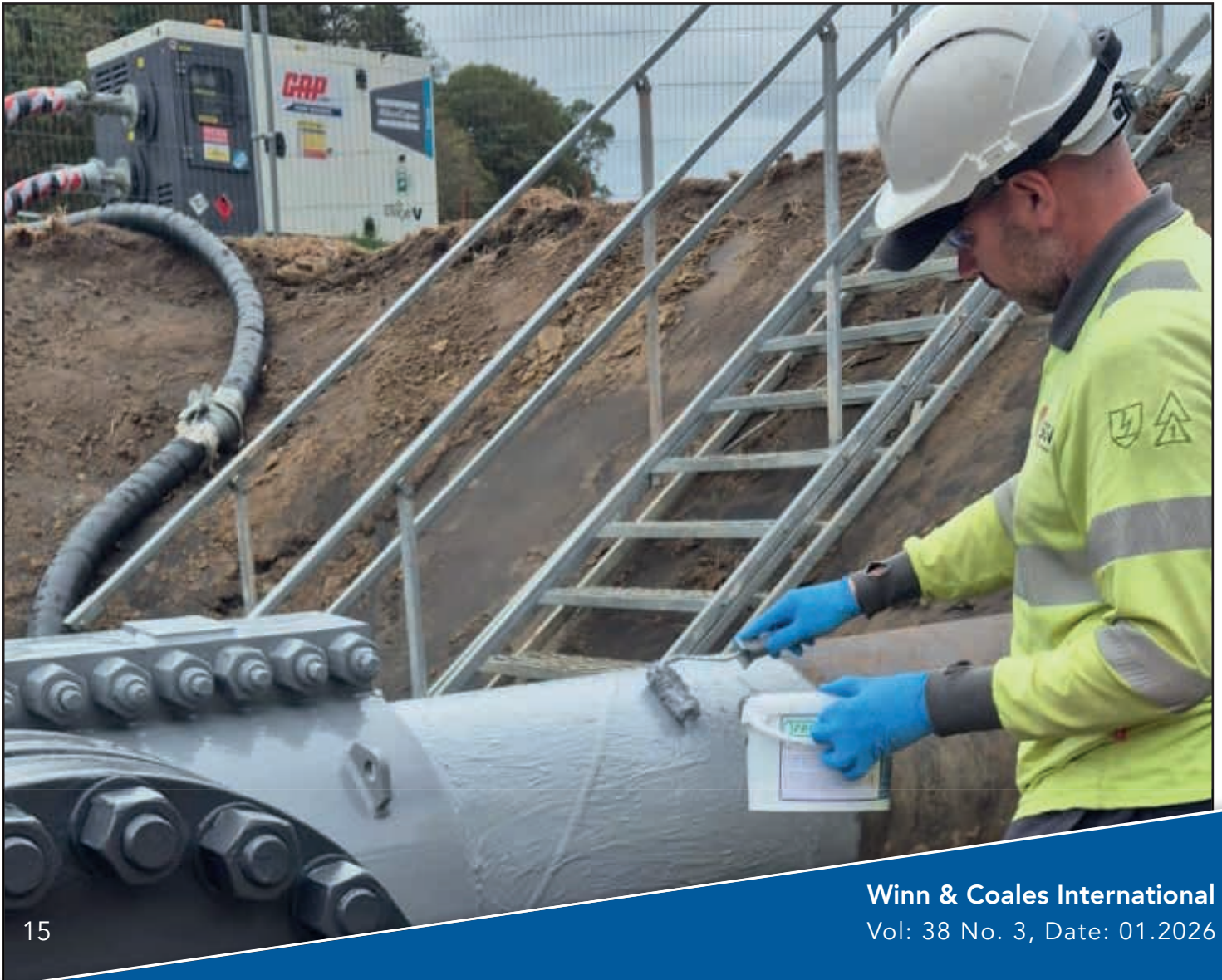
Above: Protal 7300 (UK) can be applied to dry, damp or wet surfaces. Below: Protal 7300 (UK) can be applied by roller, brush or pad.
