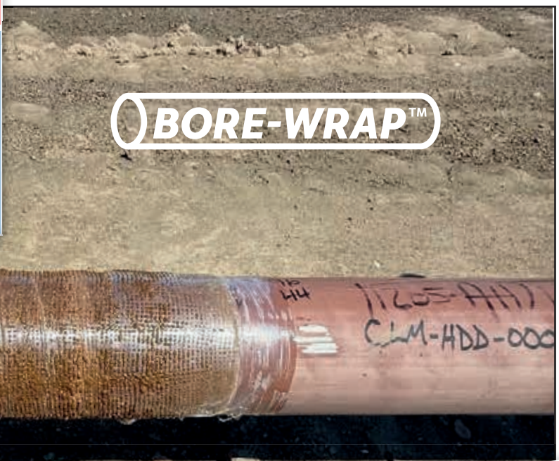
Below: Completed Bore-Wrap Application.
