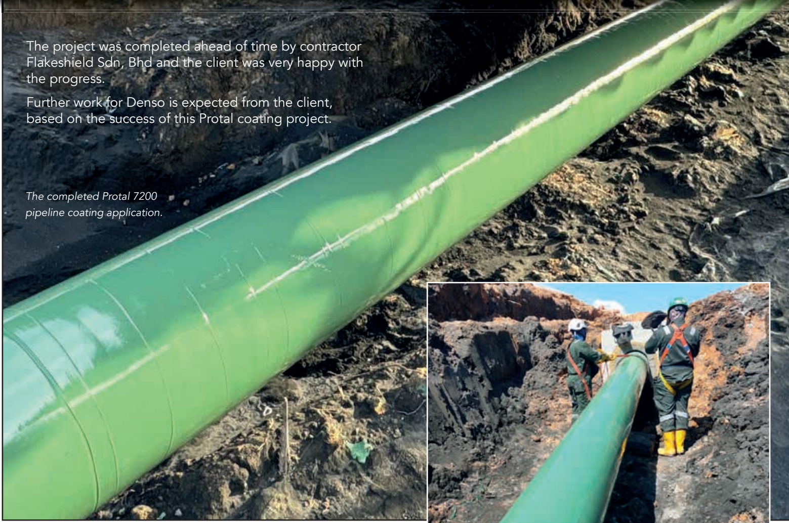
Below & right: Holiday testing of the cured Protal 7200.
