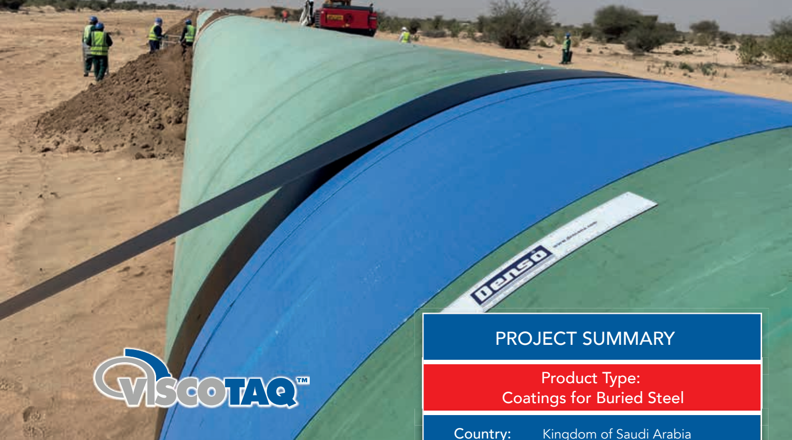
The Master Gas System Expansion Phase III in progress with girth welds receiving the Viscotaq™ HT System protection.
