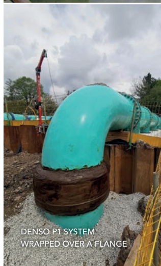
DENSO P1 SYSTEM WRAPPED OVER COUPLINGS
