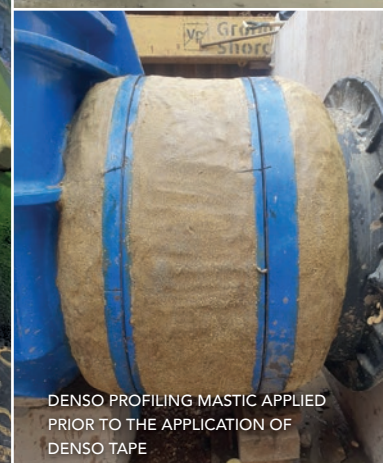
DENSO PROFILING MASTIC APPLIED TO MULTIPLE FITTINGS
