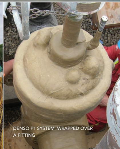
DENSO P1 SYSTEM WRAPPED OVER A FLANGE
