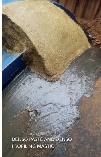
DENSO PASTE APPLIED TO PIPE, COUPLING AND NUTS AND BOLTS
