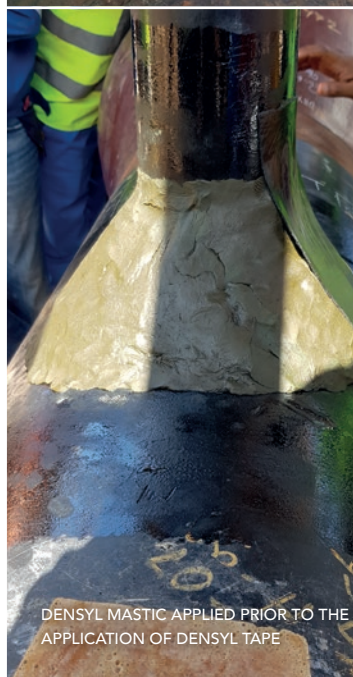
DENSO PASTE AND DENSO PROFILING MASTIC
