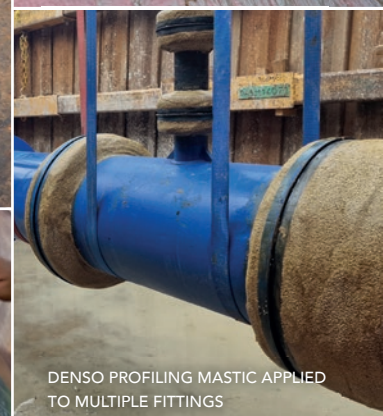
DENSO PASTE APPLIED TO PIPE, COUPLING AND NUTS AND BOLTS
