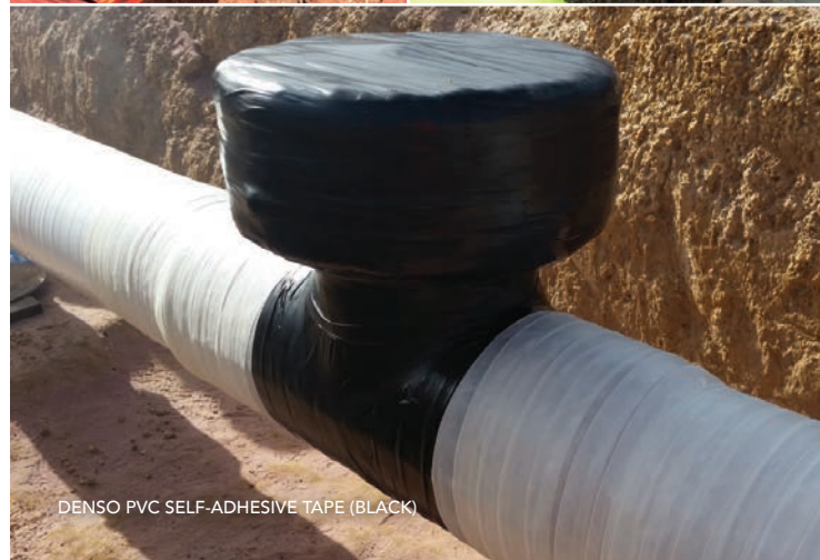
DENSOCCLAD TAPE WRAPPED OVER A FLANGE
