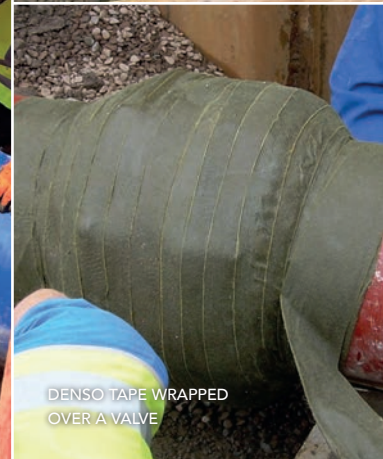
DENSO TAPE WRAPPED OVER A FITTING
