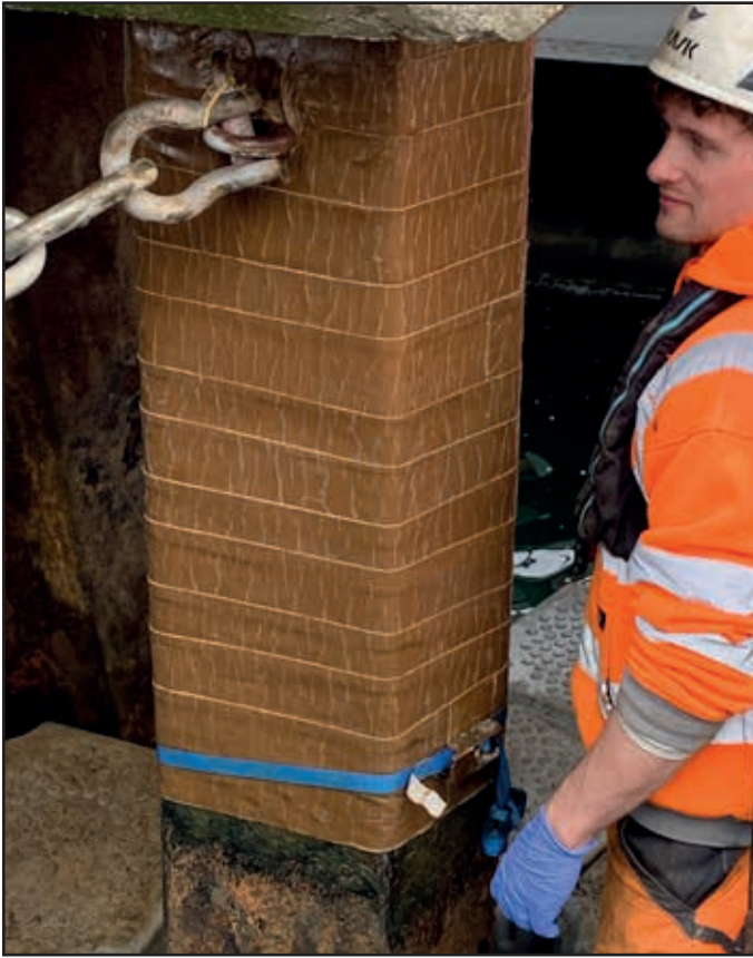
Above: A circumferential wrap of SeaShield™ Marine Piling Tape is applied to a pile (left) prior to applying the Denso™ GOW UV (right).
