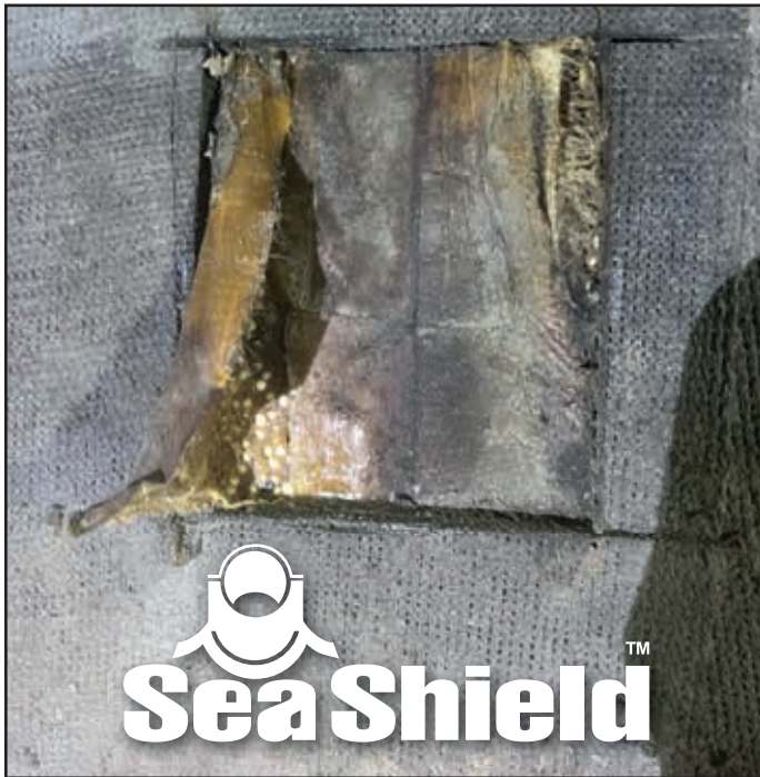
Above : A hole was cut in the 2015 applied coating and some of the Denso™ Profiling Mastic was removed to allow inspection of the inlet.
