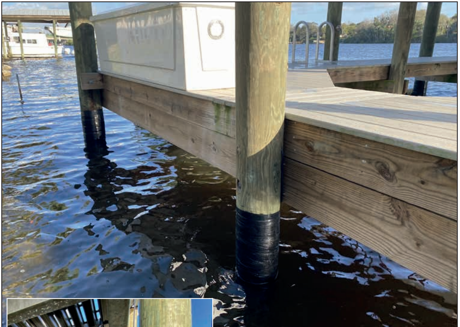
The SeaShield™ system prevents infestation of marine borers.
