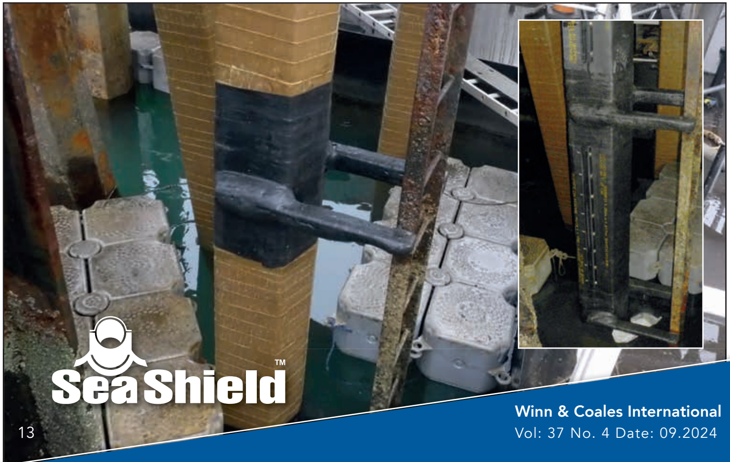
Above: A circumferential wrap of SeaShield™ Marine Piling Tape is applied to a pile (left) prior to applying the Denso™ GOW UV (right).
