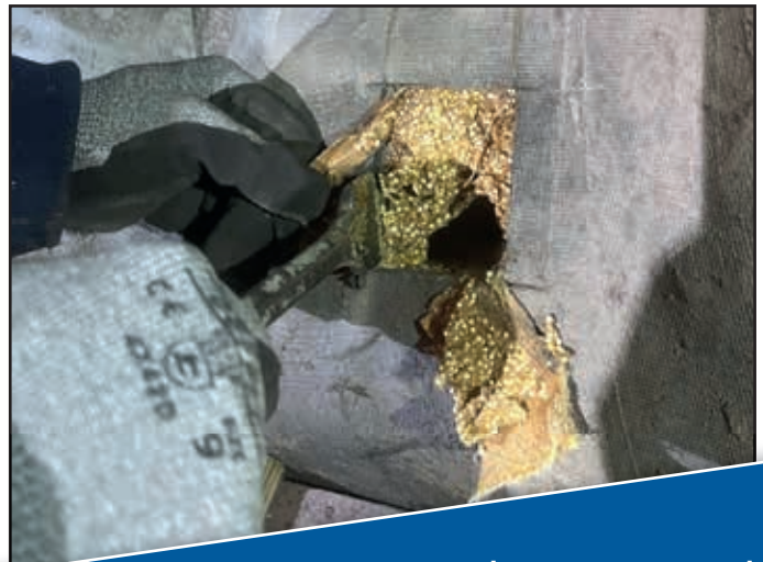
Once the inspection was complete and the inlet was found to be in good condition the Denso materials were replaced and the 2015 application was made good again.
