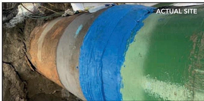
Above: The application of Viscosealant™ and Viscomastic™
