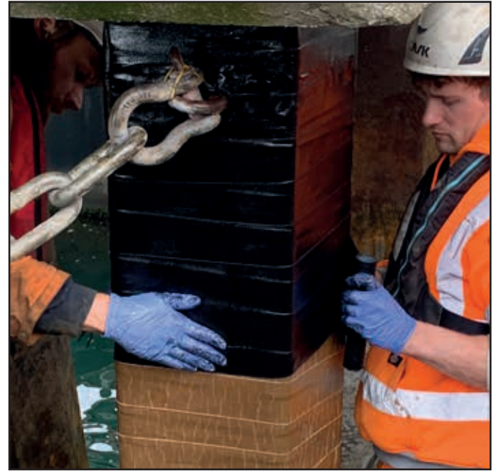
Below: Tape application complete and inset showing the completed combination of the SeaShield 2000FD™ and SeaShield 70™ Systems.
