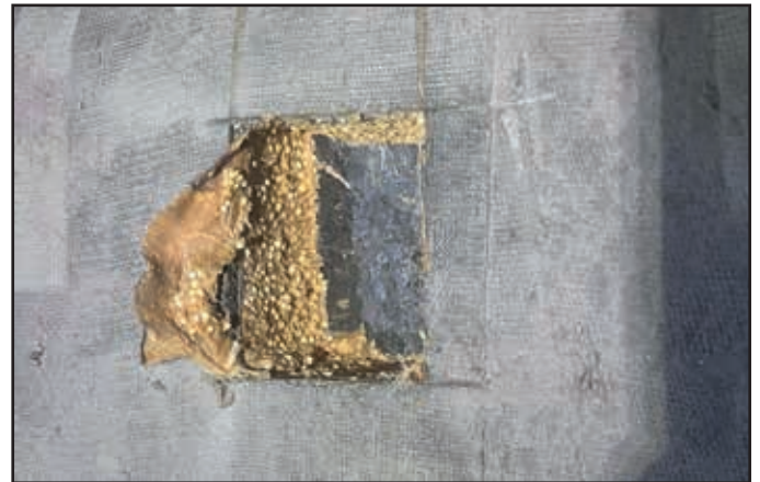
Once the inspection was complete and the inlet was found to be in good condition the Denso materials were replaced and the 2015 application was made good again.
