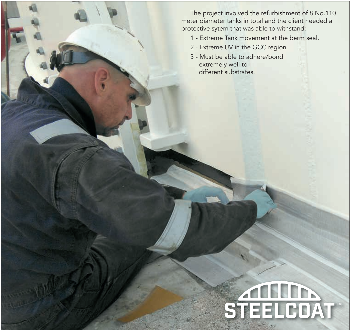
Above: The layer of Denso™ Ultraseal RT Tape is carefully fitted into place before a coat of Denso Acrylic Topcoat is applied over it to complete the Denso Steelcoat System.
