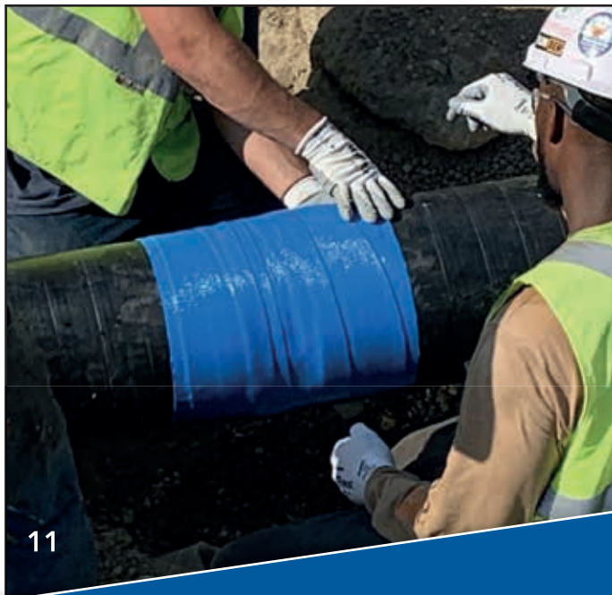
Below and right: The completed ViscoWrap XHT joint protection.
