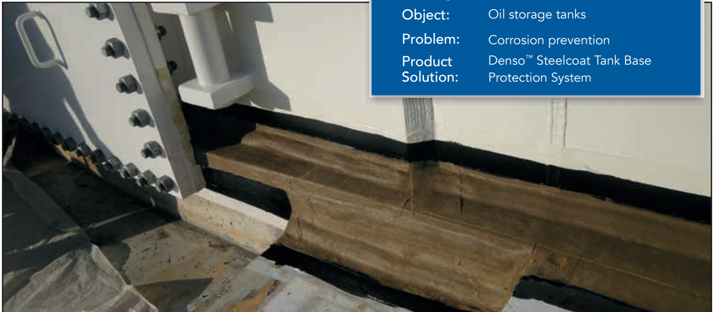
Above: After cleaning the substrate around the berm seal area and coating it with Denso™ Hi-Tack Primer, any voids or internal angles are filled with Densyl™ Mastic to form a smooth profile before applying the layer of Denso™ Hi-Tack Tape. Then Denso Primer D™ is applied to the area immediately around the Denso Hi-Tack Tape in a minimum 50mm strip and allowed to dry (Primer D is the black area in the picture).
