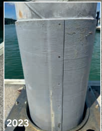
View of the SeaShield 500 Jacket showing its vertical overlapped joint.
