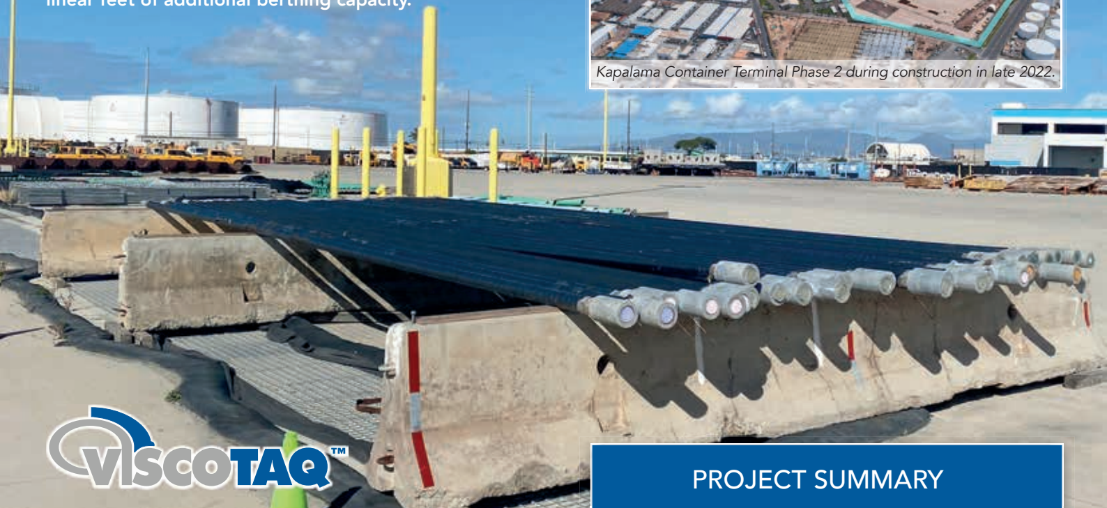
Above: Tie rods wrapped with Denso™ Tape followed by a Viscotaq™ PVC Outerwrap.
