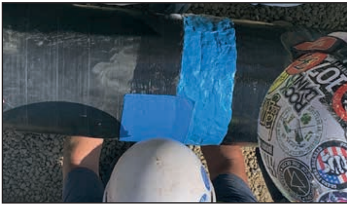
Below and right: The completed ViscoWrap XHT joint protection.
