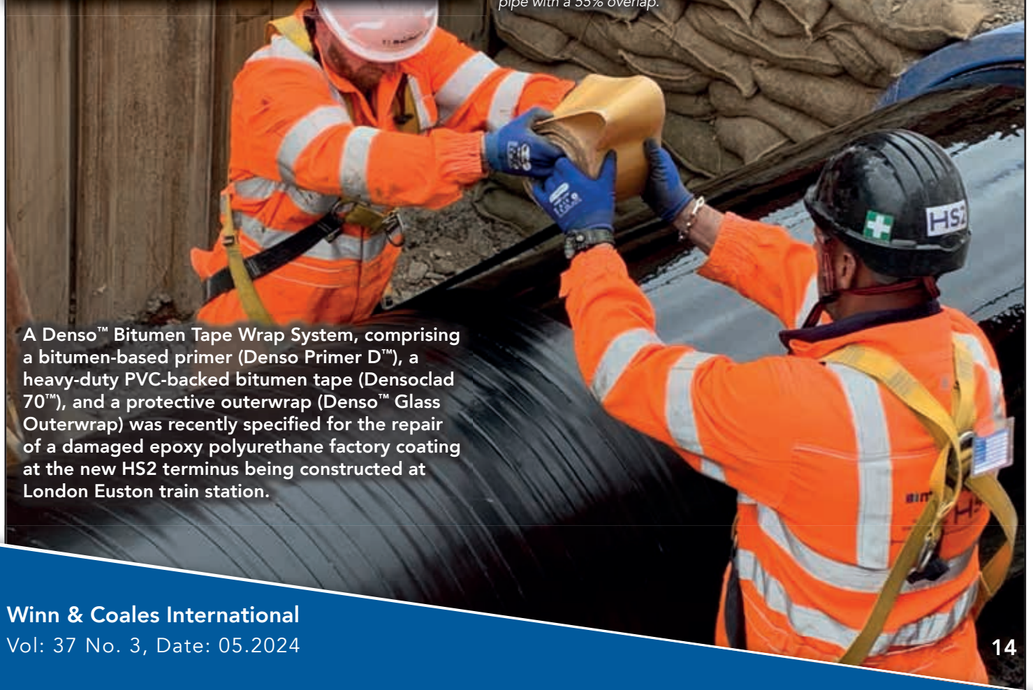
Below: Densoclad 70 is then circumferentially wrapped around the pipe with a 55% overlap.
