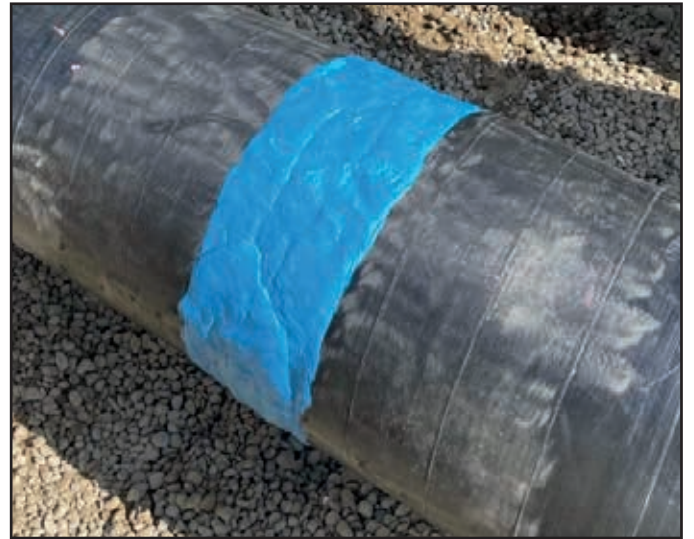
Applying the ViscoMastic XHT to smooth the joint's profile.
