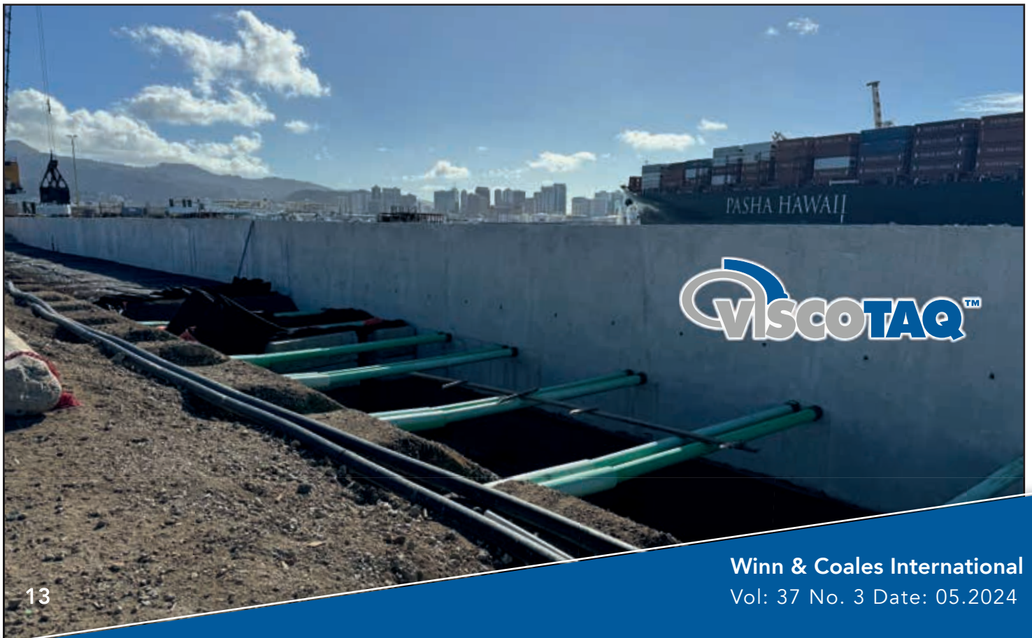
Above: The Denso™ wrapped tie rods are first installed and then...Below: Protected with PVC piping before final burial.
