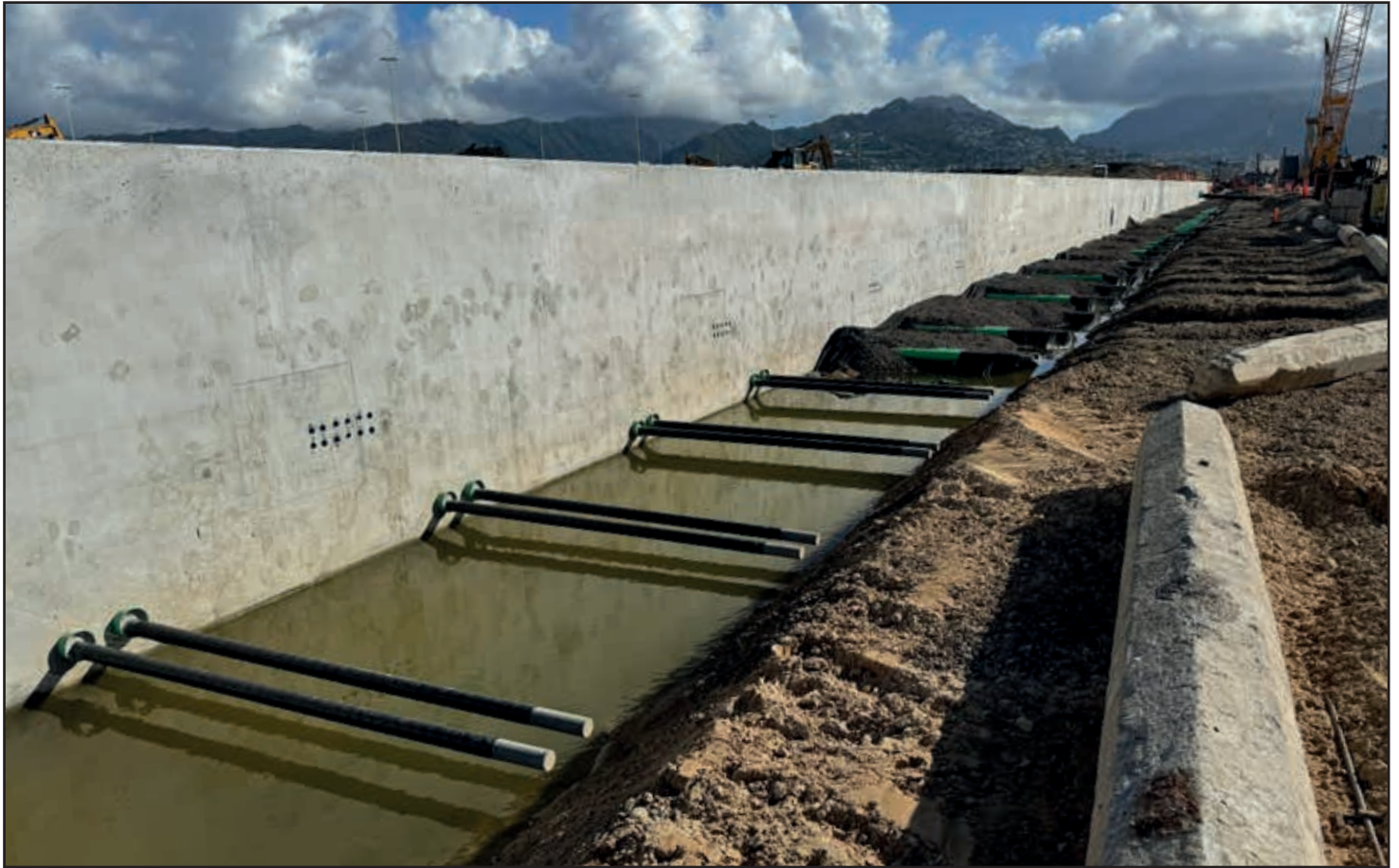
Above: The Denso™ wrapped tie rods are first installed and then...Below: Protected with PVC piping before final burial.
