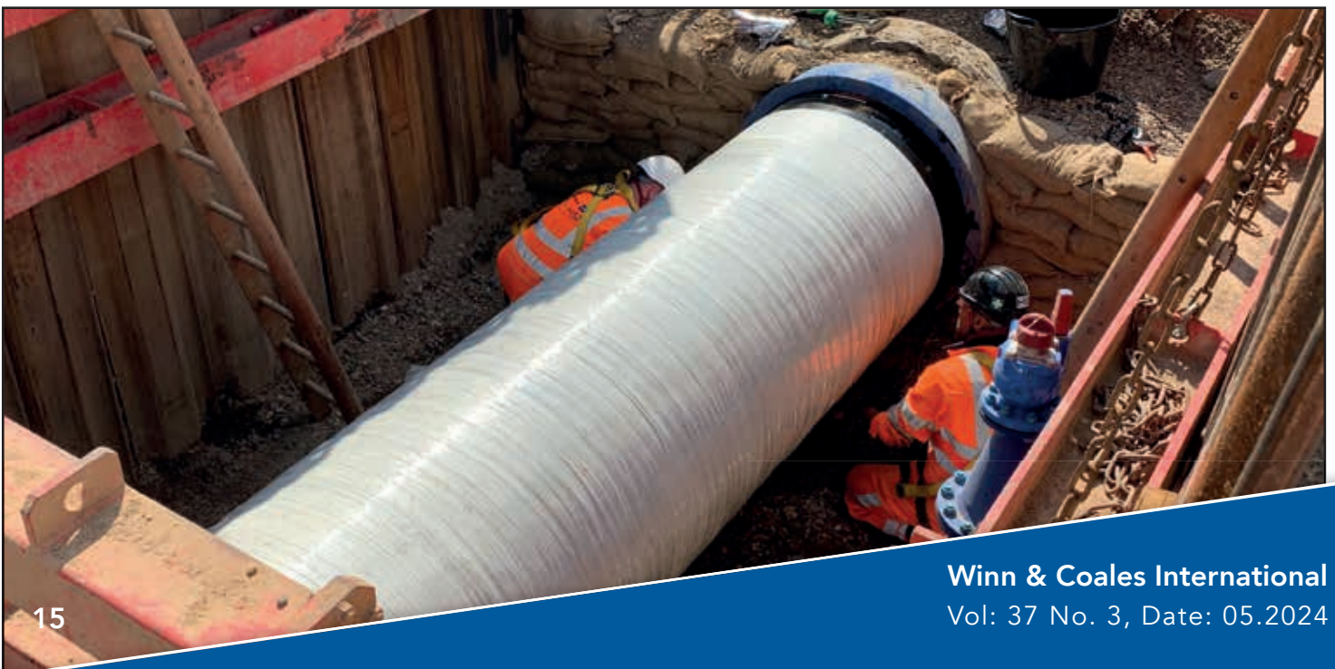
Below: Completed application of Denso Glass Outerwrap.
