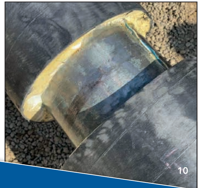
The field weld area after surface preparation.
