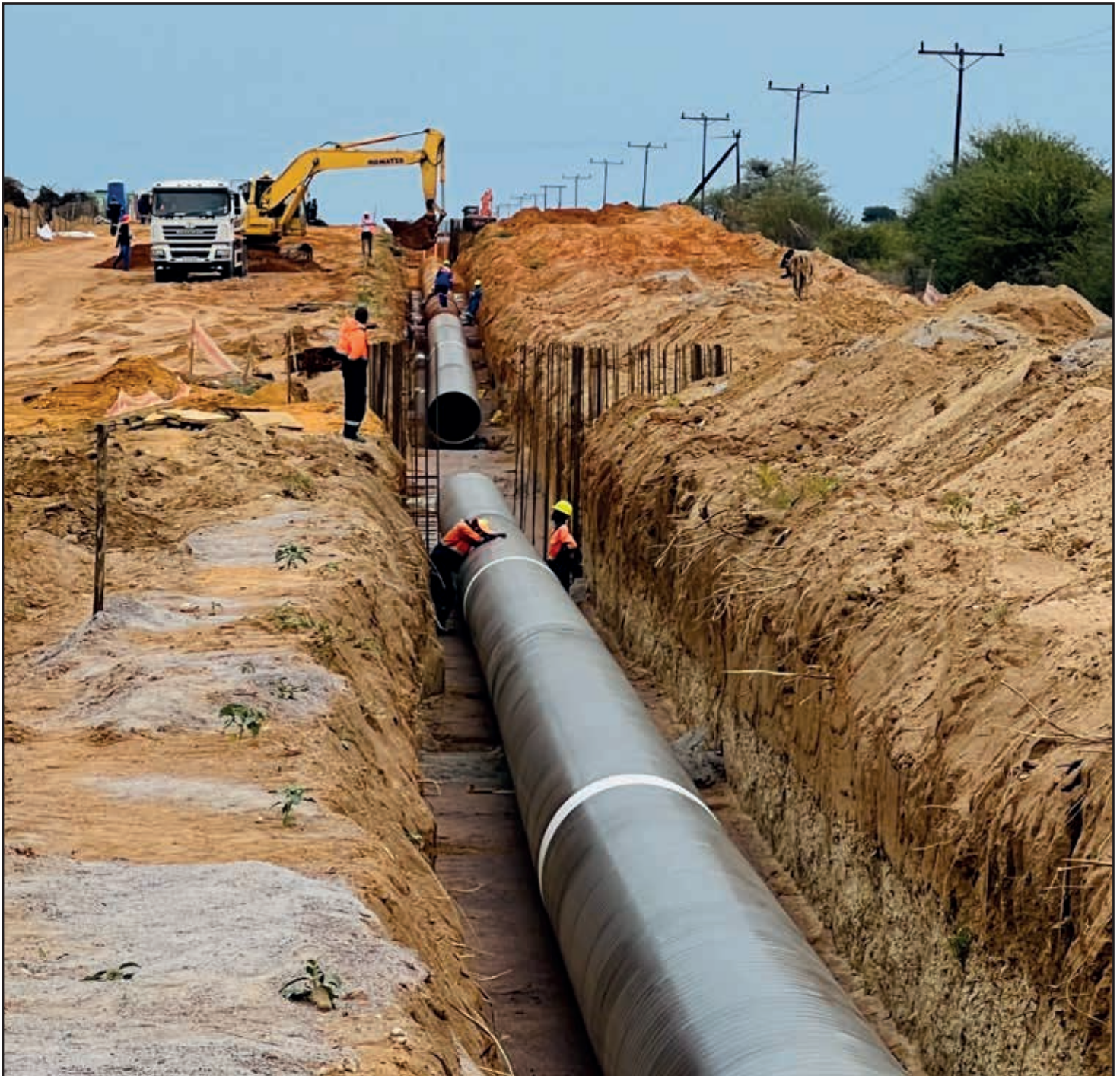
Excavator backfilling once the pipeline has been installed and inspected for any damages..
