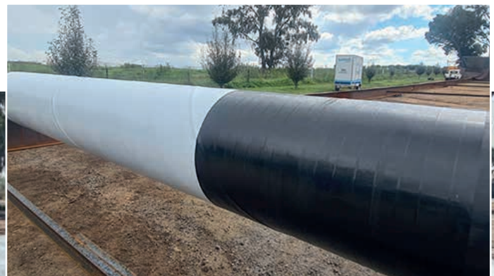
Inset: The Denso Butyl Tape System comprises Denso S43™ Innerwrap followed by Denso R23™ Outerwrap.
