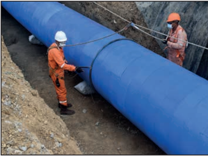
Holiday detection equipment used for routine check.
