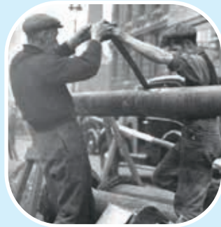
Early Densotherm and Denso Tape applications.
