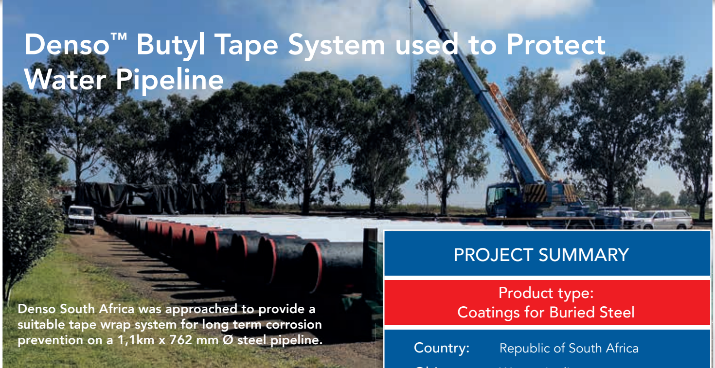
Above and below: Butyl Tape wrapped pipes awaiting installation.
