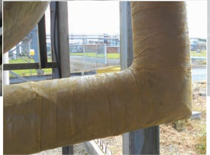
Above: First, Denso Hi-Tack Petrolatum Tape is applied to the pipe.
