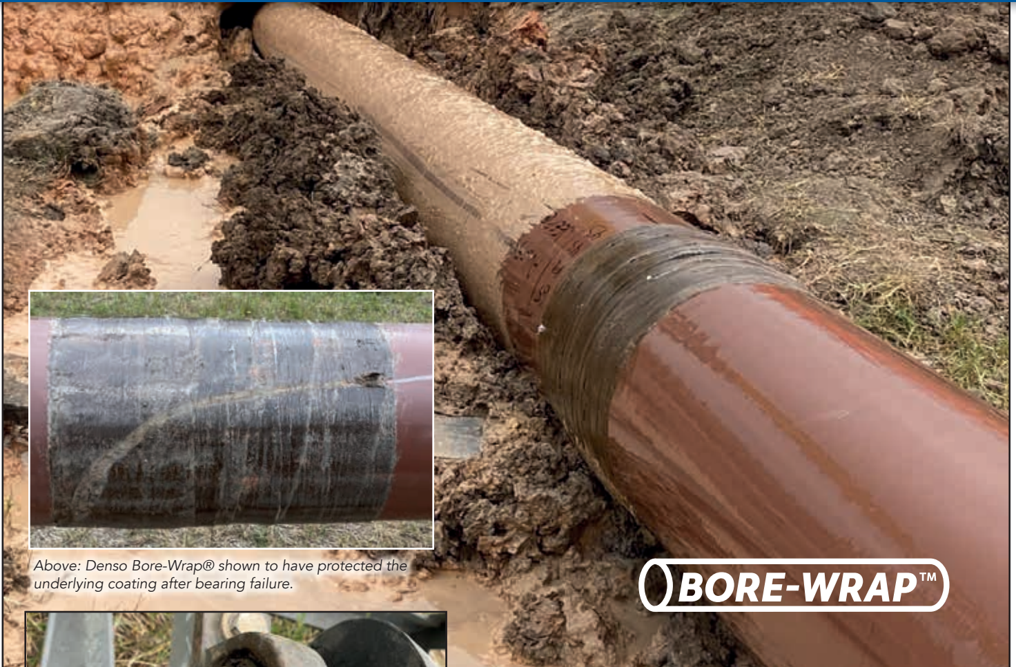
The first weld joint after exiting the bore hole.
