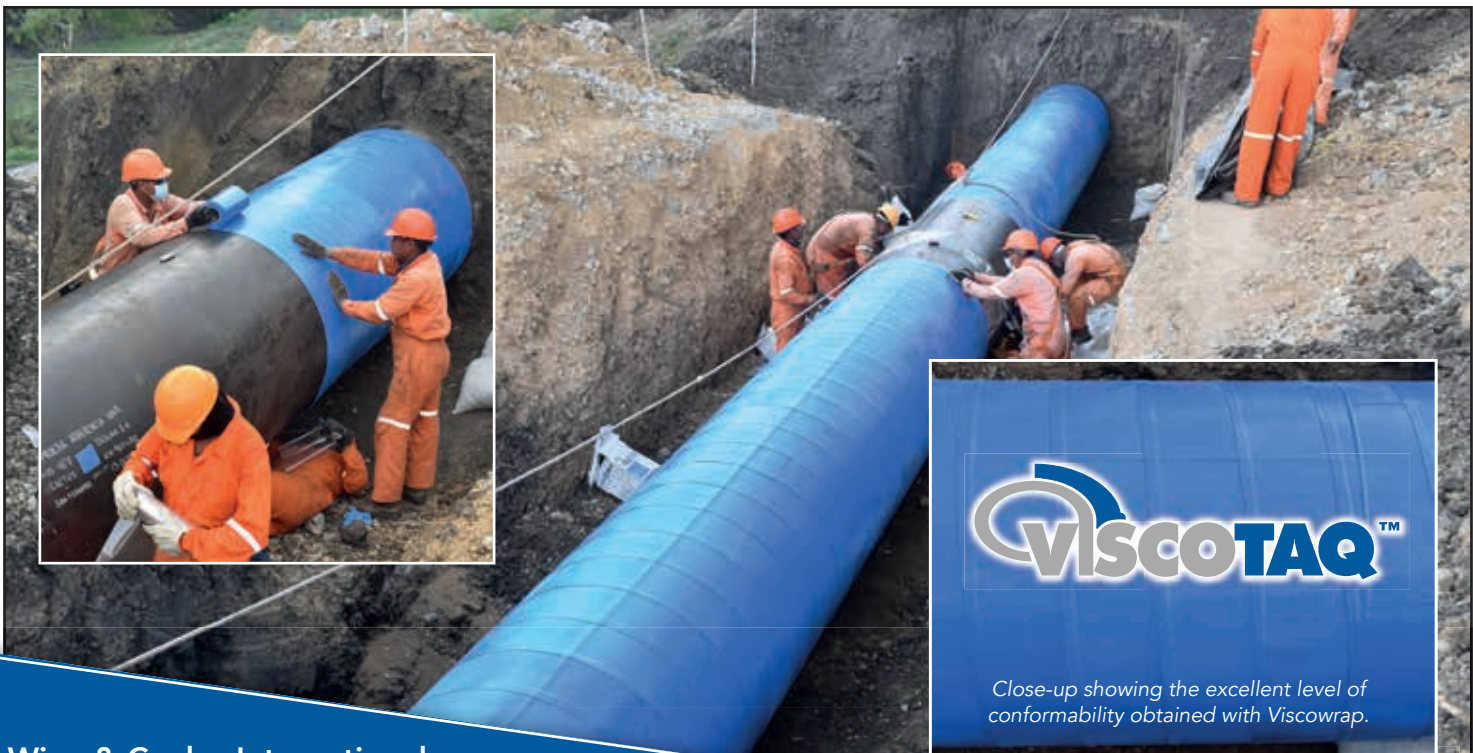
Below: The application of the Viscowrap inner Layer.
