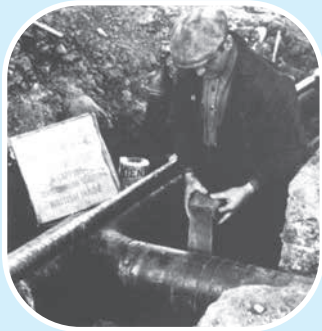
Early Densotherm and Denso Tape applications.
