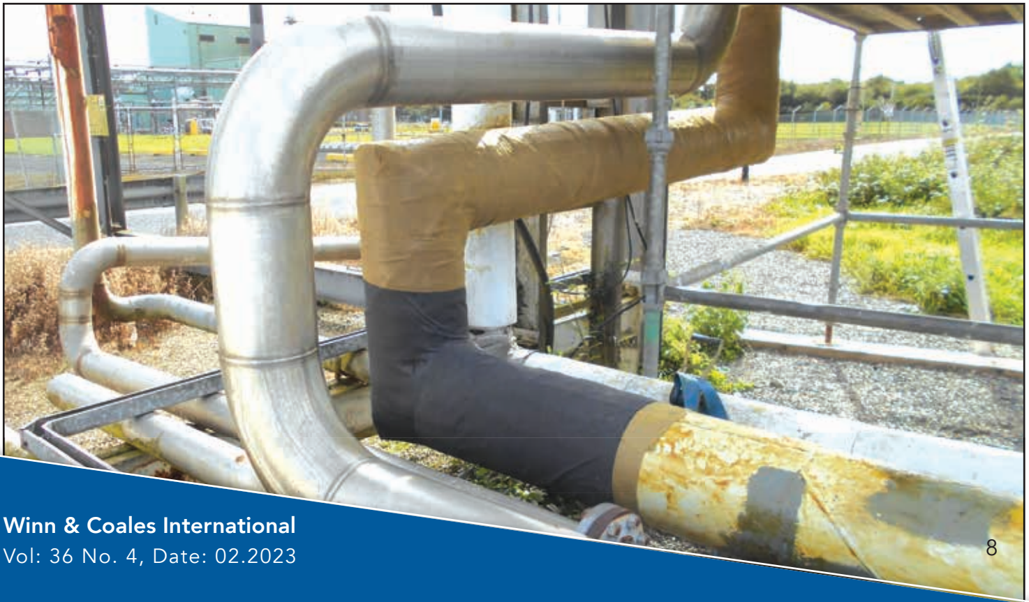
Below: Denso Ultraseal Tape is then applied over the Hi-Tack Petrolatum Tape.
