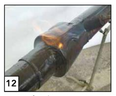
Beginning from the center again, lead the flame to the closing strip in circumferential direction, while shrinking the spigot end.
