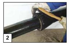
Clean the pipe surface thouroughly to very thouroughly (St 2 - St 3) with a hand wire brush. Remove rust, dirt and other residues.
