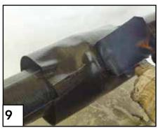
Apply the same procedure for the other side of the closing patch.
