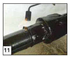
Press the sleeve while warm to ensure full contact with the pipe. The shrinking procedure is finished when the sleeve fits tighly and the thermo-indicator is no longer tangible.
