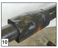
Beginning below, warm the shrinkable sleeve in the middle, moving the torch in a circumferential direction with blue-yellow flame. Next, shrink the spigot side using the same motions. Finally, shrink the socket side. Ensure even shrinkage.
