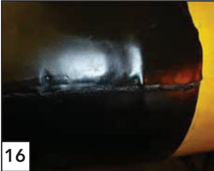
16 A bead of extruded butyl rubber is visible at the edge of the sleeve.
