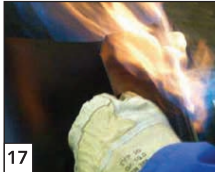
17 Warm one end of the adhesive side of the closure patch with a gas flame. Position the warmed side of the closure patch over the exposed edge of the sleeve.
