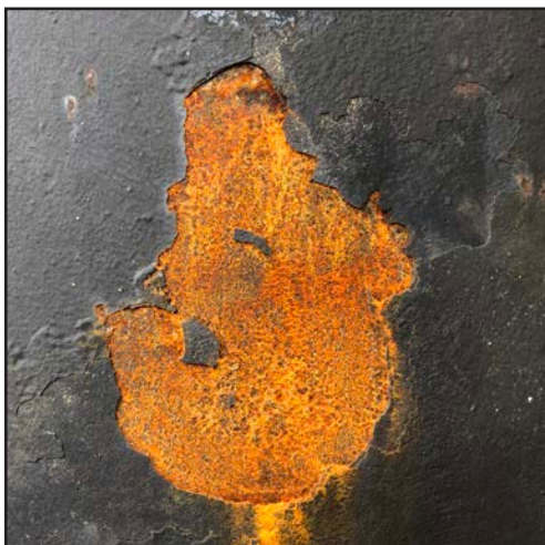
Example image showing tightly adhering corrosion prevention coating and corrosion (orange rust) that would not require removal.
