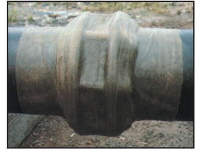
Completed coupling
