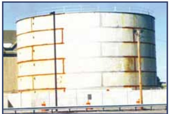
Above: Foremost area of Tank is treated with HoldTight 102. Flash rust is clearly visible either side of where the HoldTight was applied.
