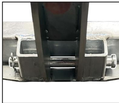
Fig. 3: Clamping Bar fitted correctly with clevis pin
