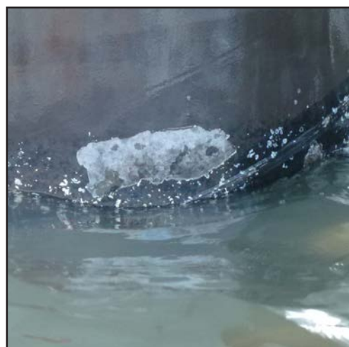
Example image of a pile featuring acceptable levels of non-living, tightly adhering mineral deposits.
