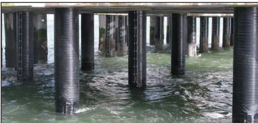
The SeaShield 250HD system installed on the gas transmission platform support piles.
